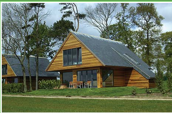
Cedar Lodges – K P Club, Kilnwick Percy, East Yorkshire Cedar used for cladding luxury cabins
