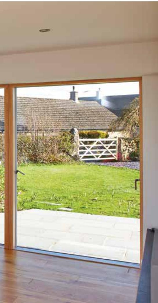
the building. Echoes of the slate roof are found in the black limestone paving and even the slate hearth inside. The Velfac window system fits with the house's contemporary style, with anthracite frames on the outside to match the flashing, and pine interiors.
